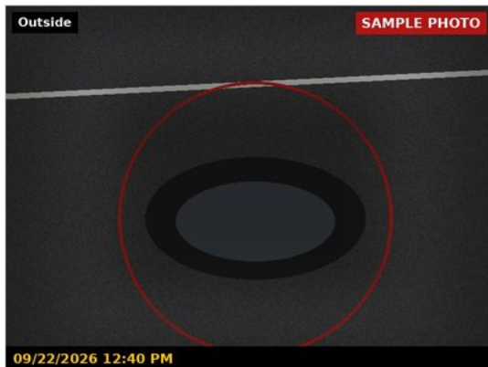
Pothole - Building E row
