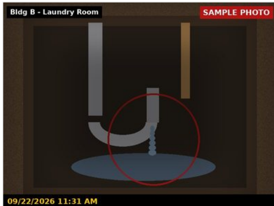
Leak at washer supply
