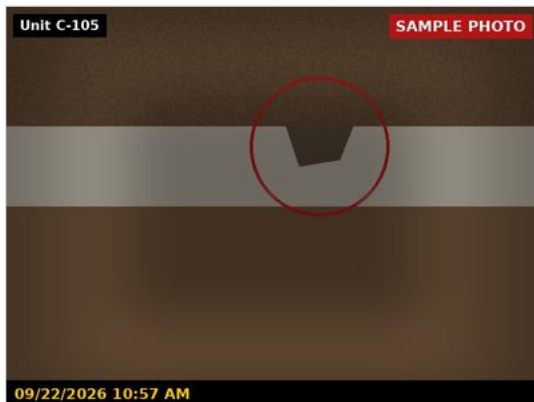
Countertop damaged at sink
