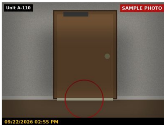
Weatherstripping missing
