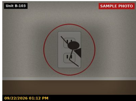
Cracked receptacle
