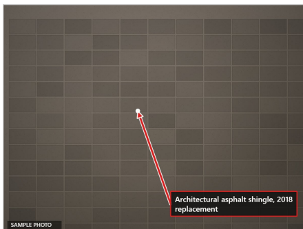
Architectural asphalt shingle, 2018 replacement
