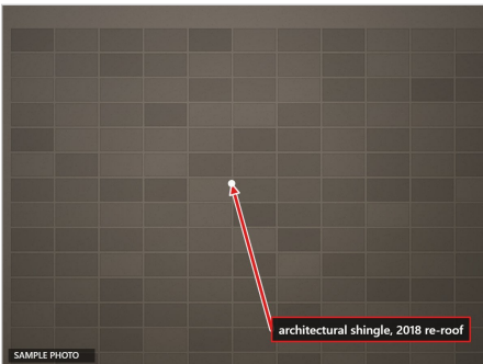
South slope - architectural shingle, 2018 re-roof (1 of 4)
