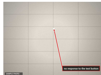
Hallway smoke alarm - no response to t
